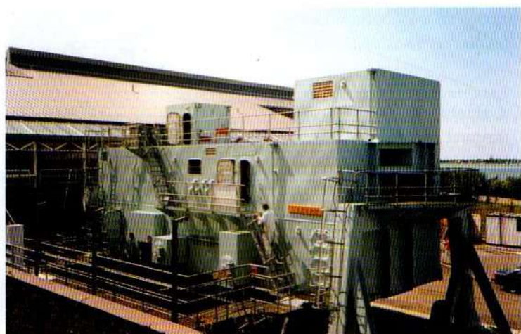
Figura 2- Damage Repair Instructional Unit
